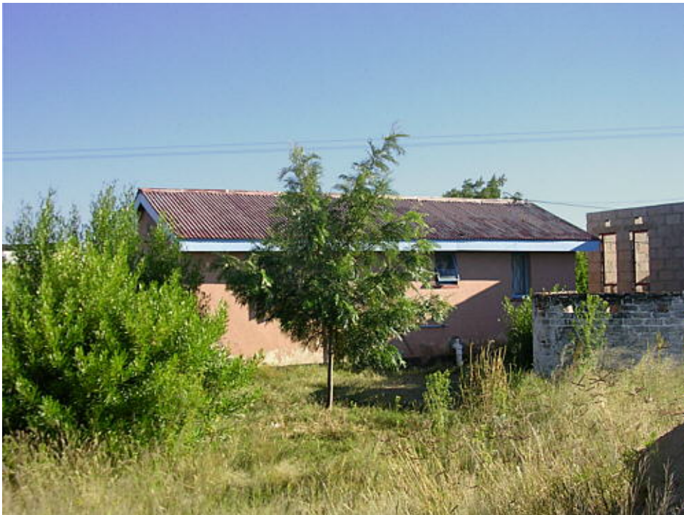
View of the south-by-southeast corner of the house and plot
